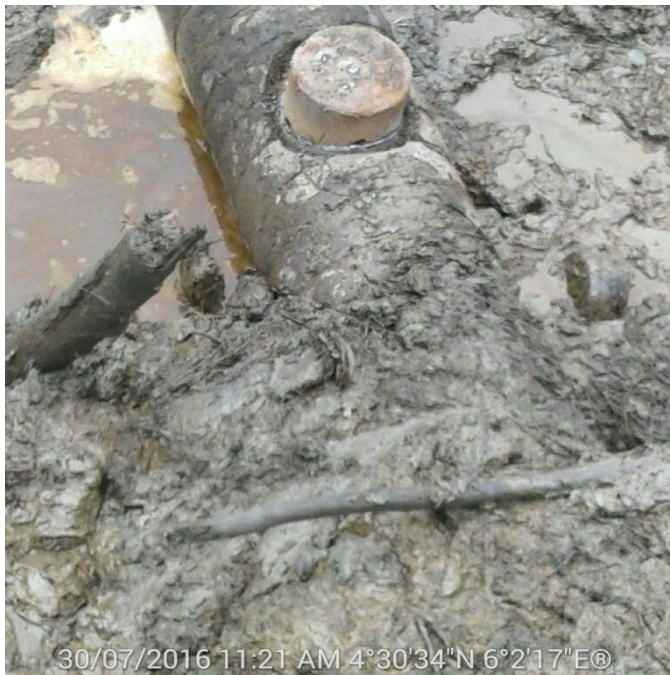
Fig F: Incident Facility during repair
