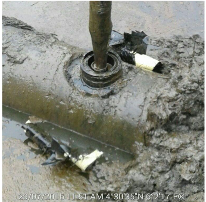
Fig E: The spill point after excavation
