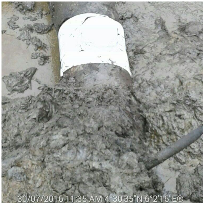
Fig G: Incident Facility after repair
